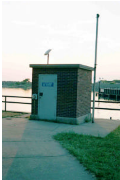
Figure 3.15. Cleveland gauge house.
